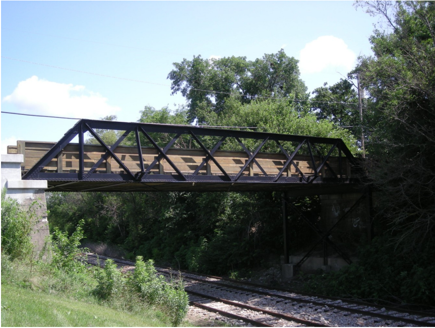
Steel Truss, Quadrangular Warren bridge
