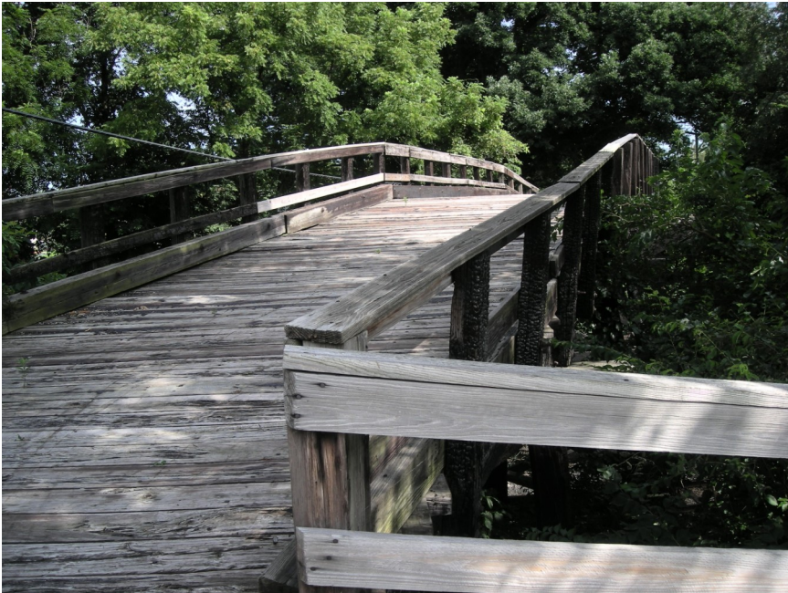
Timber Stringer bridge
